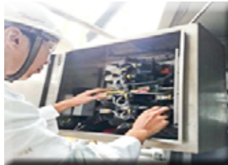
Electrical Insulation Check
